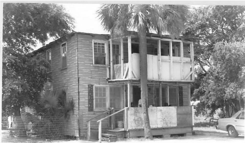
Pine Tree Hotel (July 1989) – Pre Hurricane Hugo
